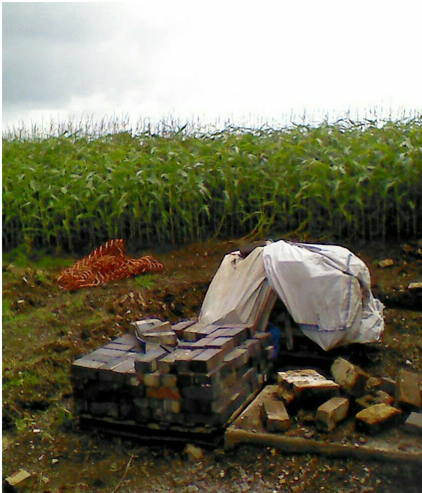
Materials on site awaiting use.
