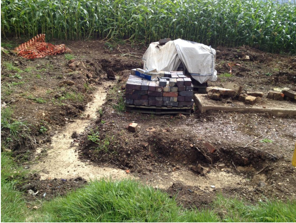
Footing dug and laid
